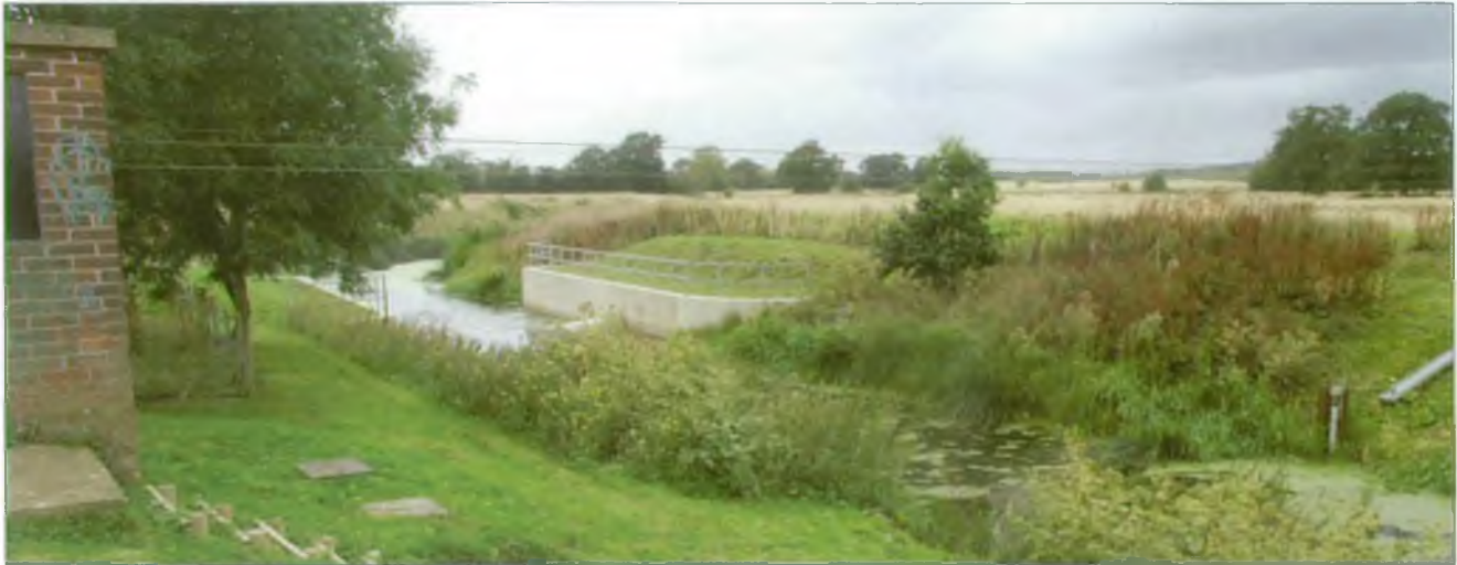
This gauging station is at Stilebridge on the River Beult. In CAMS we use flow data to calculate benchmark flow
