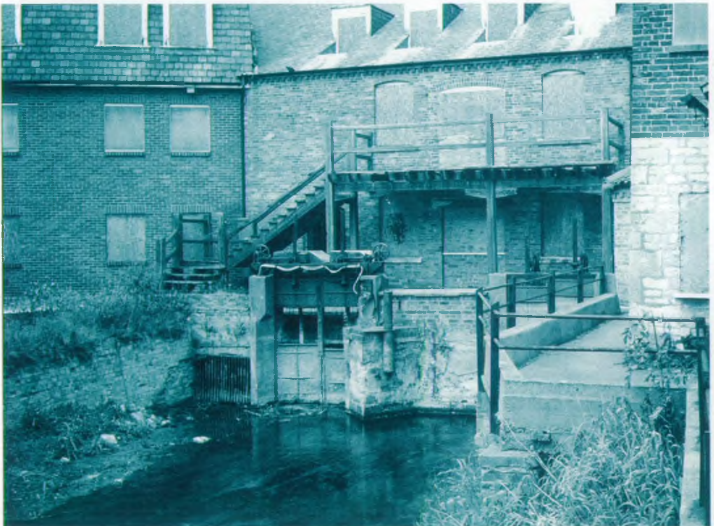
Navigation structure impeding fish pass
