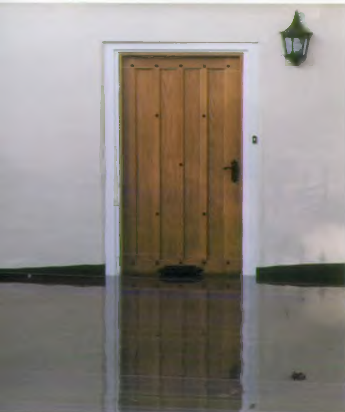
▼ Shrewsbury floods - November 2000
