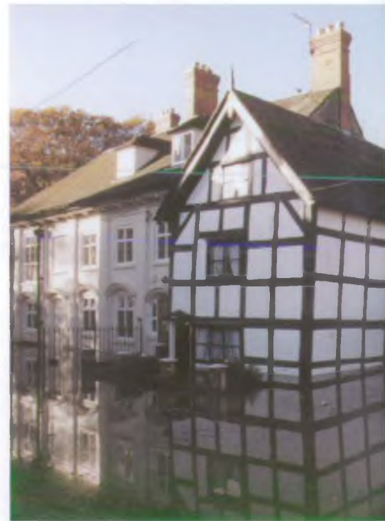
▲ Shrewsbury floods - November 2000
