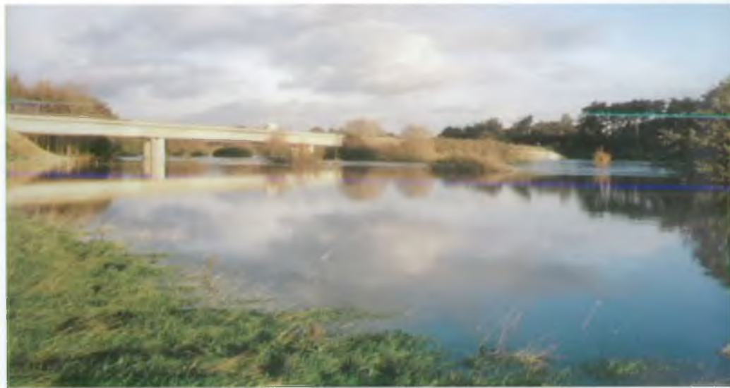
▲ Shrewsbury floods - November 2000
