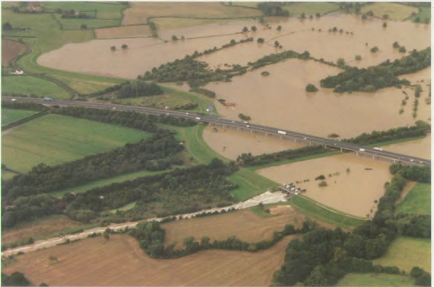
Leigh barrier, holding back flood water - photo by Environment Agency
