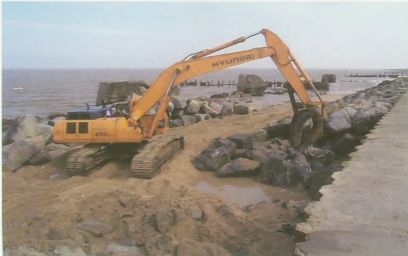
Repairing flood defences at Bulverthythe - photo by Environment Agency
