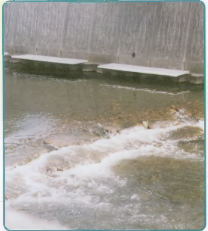
The recently constructed weir at Bridgend ▶
