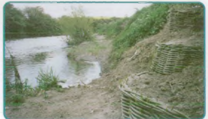
Bank erosion control for North East Region for the Kilnhurst Project ▷ △
