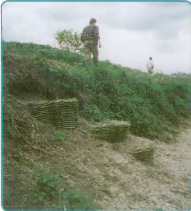
Bank erosion control for North East Region for the Kilnhurst Project ▷ △
