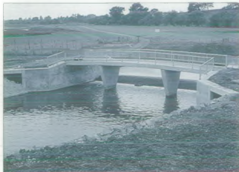
Haversham Weir, looking upstream.
