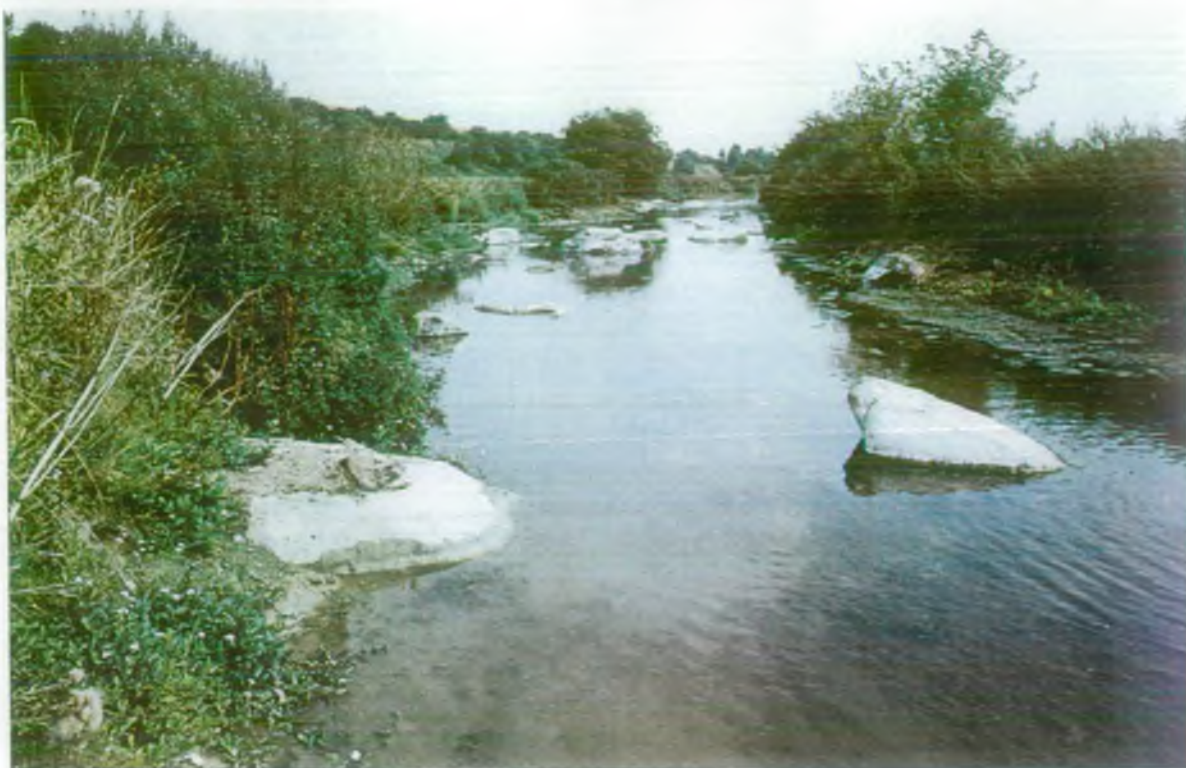
Plate 15: Kennet downstream of Fyfield Church. Sarsen stone groyne enhancement works (1.9.93)
