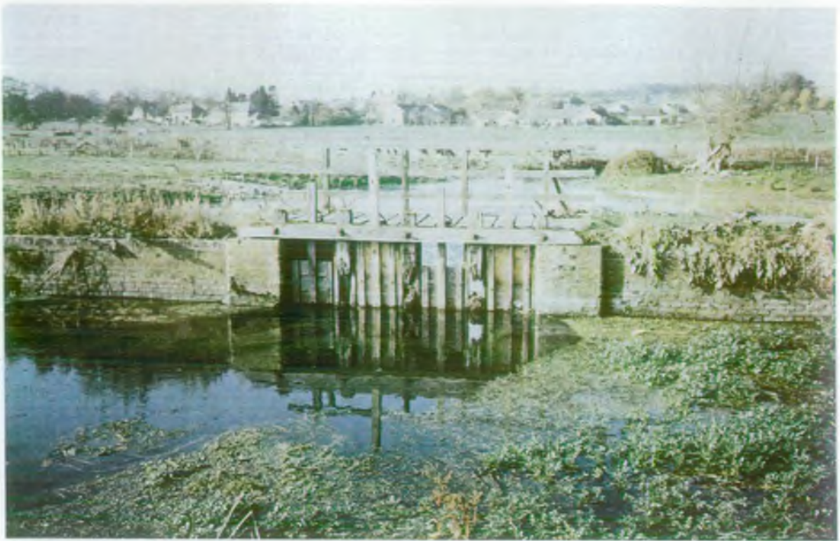
Plate 26: Kennet immediately upstream of Mildenhall hatches (4.11.93)
