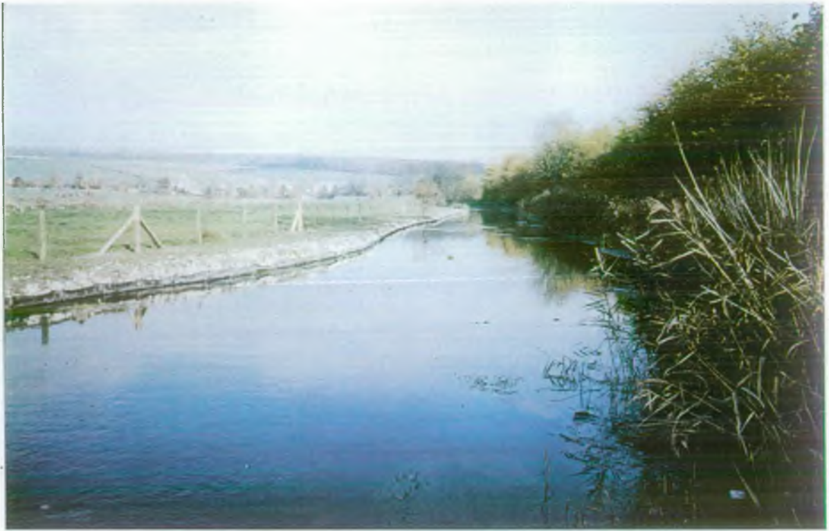
Plate 22: Kennet; channel narrowing works upstream of Mildenhall hatches (4.11.93)
