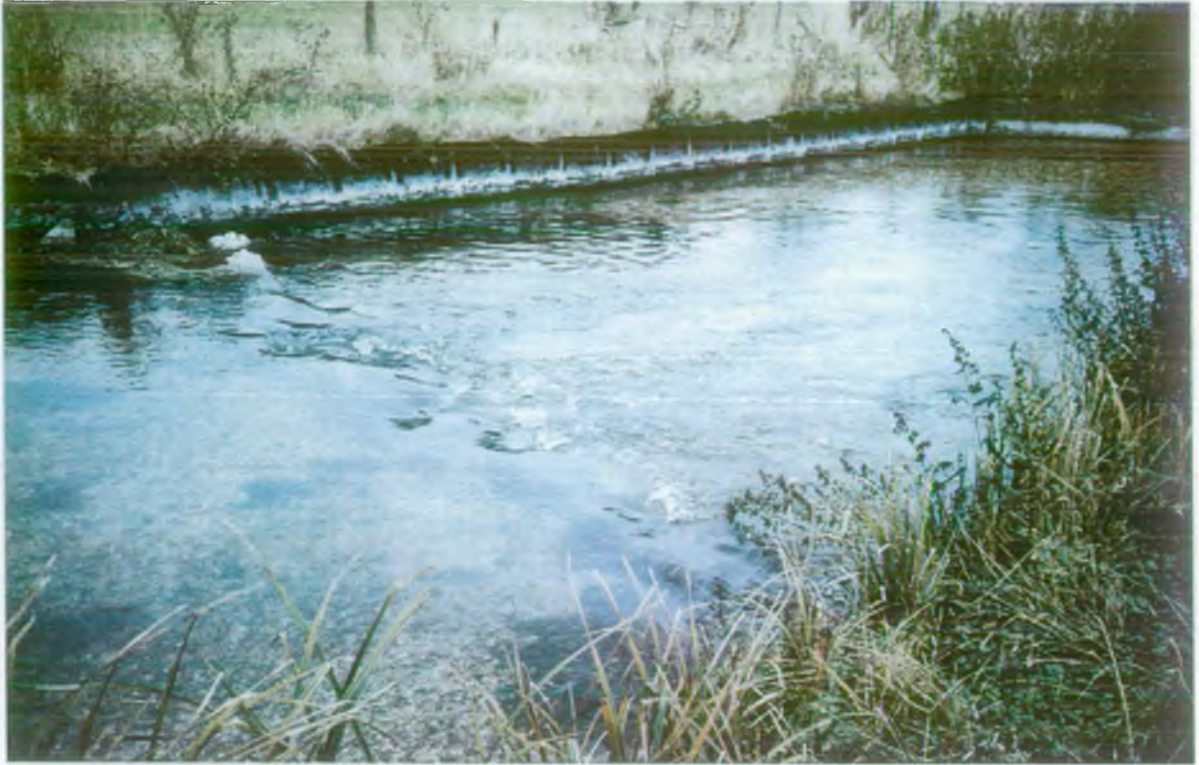
Plate 32: Kennet; channel narrowing and weir construction downstream of Rags Hatches, Axford Estate (4.11.93)
