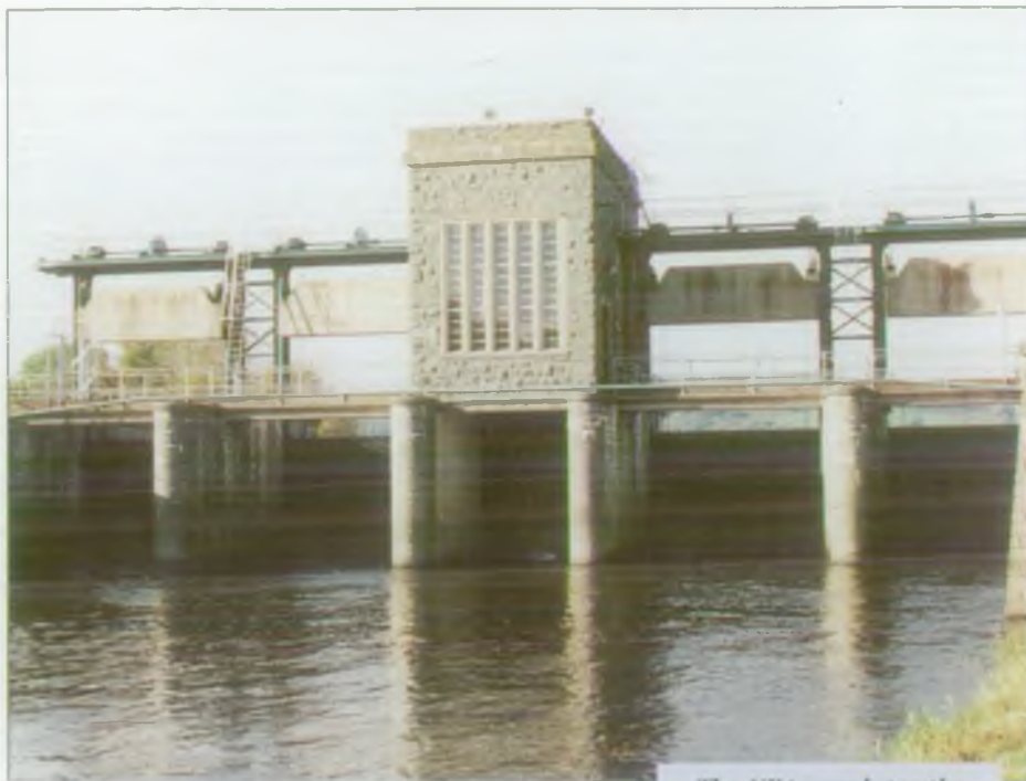
The NRA regulates the river Dee by operation of the Bala sluices.
