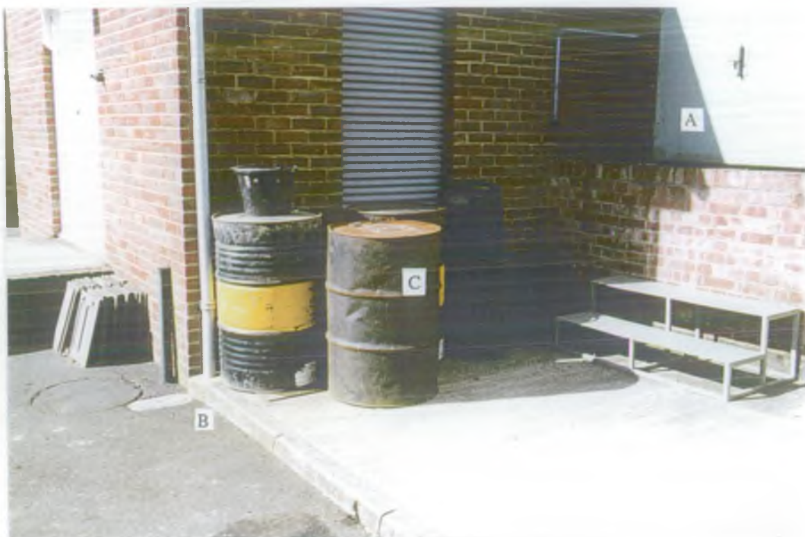
Picture 5 Leigh Office fuel dispensing area and drums stored alongside bulk oil tank. A - fuel dispensing point; B - unsealed rain water downpipe; C - oil drums.
