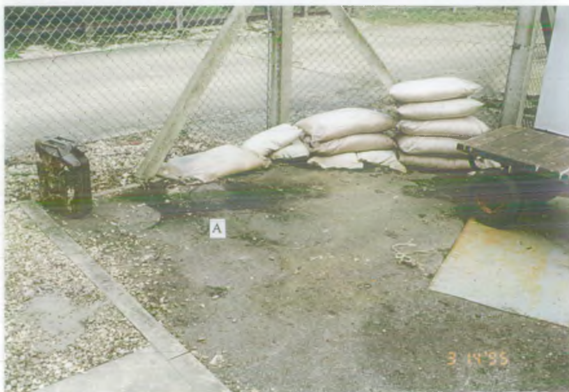
Picture 6 Leigh Office unbunded store area alongside Portastore building. A - marks due to oil spillage and drums.
