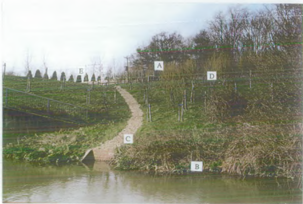
Picture 2 Leigh Office and barrier with Powder Mill Stream in foreground. A - sewage treatment plant; B - sewage outfall; C - land drain; D - tree planting scheme; E - Leigh Office.
