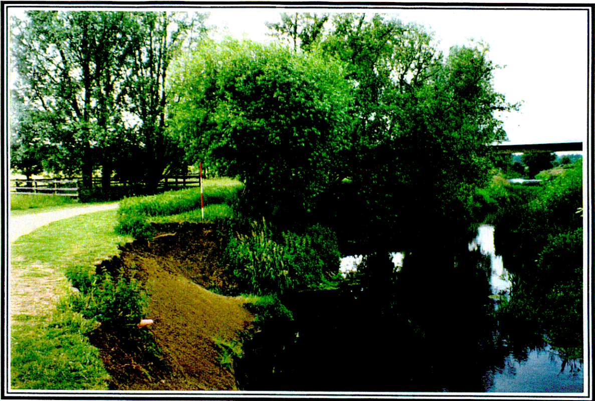
Plate 3: River Ouzel (Milton Keynes Valley Park) - traditionally pollarded willow in the foreground with un-pollarded, yet mature, willows beyond. Note the extreme erosion before the pollarded willow, and under the un-pollarded willows. Note also the difference in herbaceous vegetation diversity between the willows
