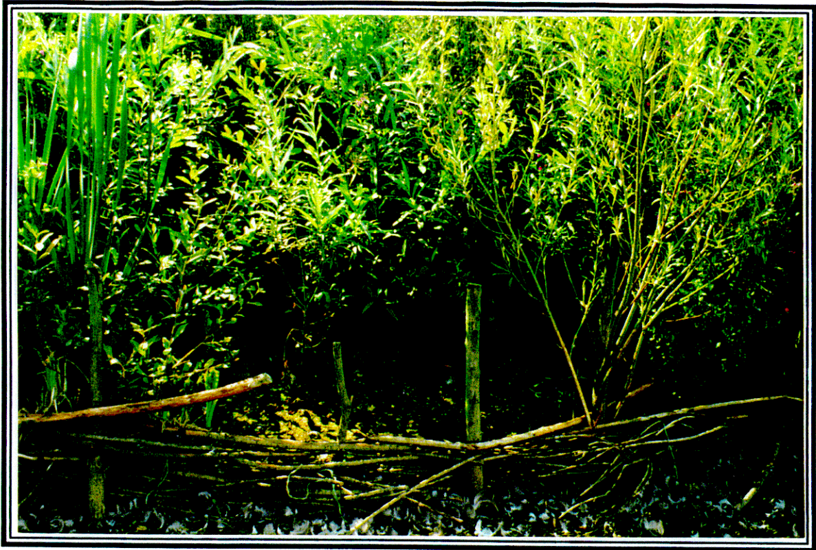
Plate 27: River Great Ouse (Milton Keynes) - note the willow poles have grown, but the spilings have not grown. The spilings act as a barrier to continued erosion
