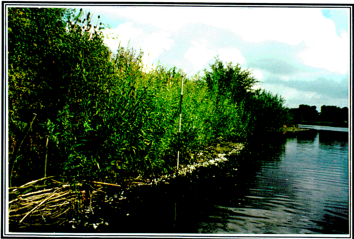
Plate 27: River Great Ouse (Milton Keynes) - note the willow poles have grown, but the spilings have not grown. The spilings act as a barrier to continued erosion
