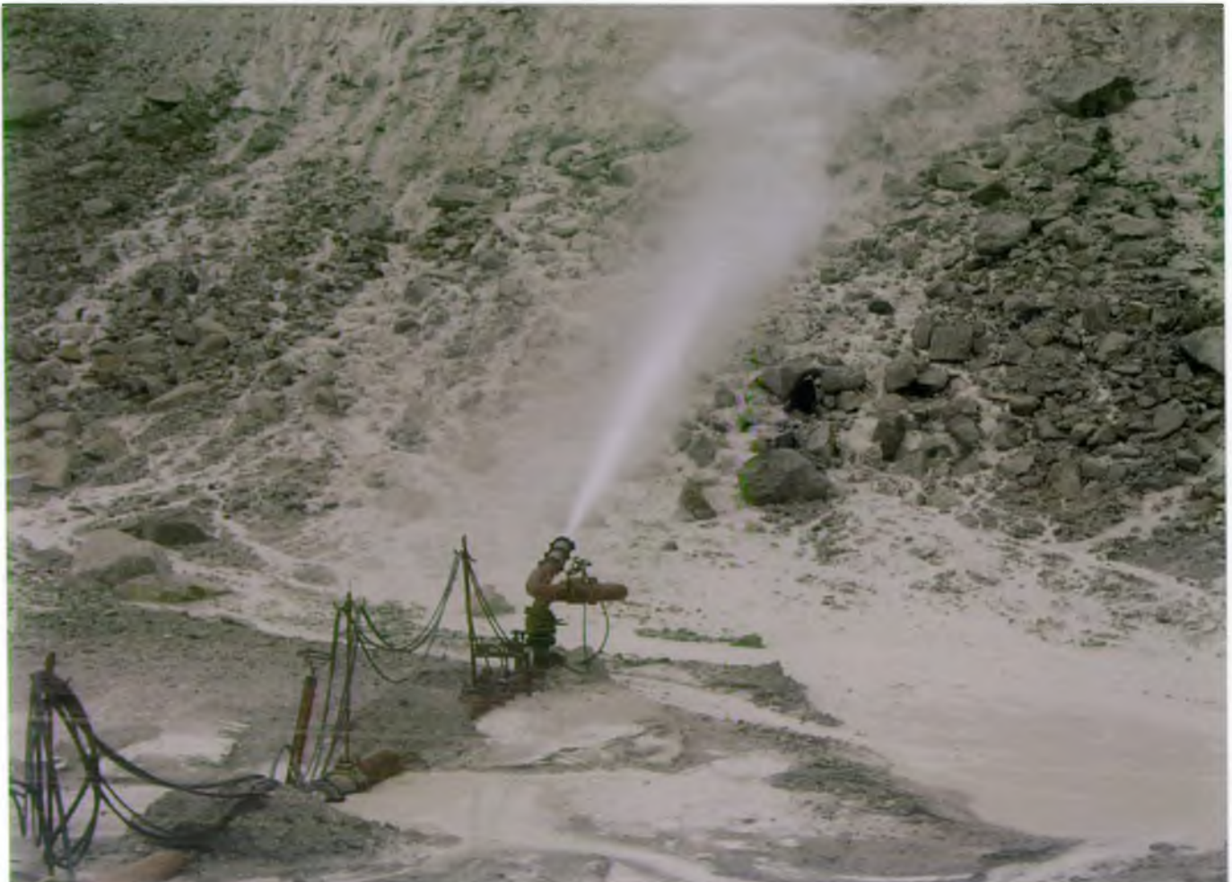
Use of water in Blackpool Pit
