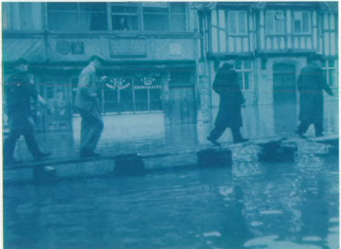
Flooding at Bewdley in the 1940s
