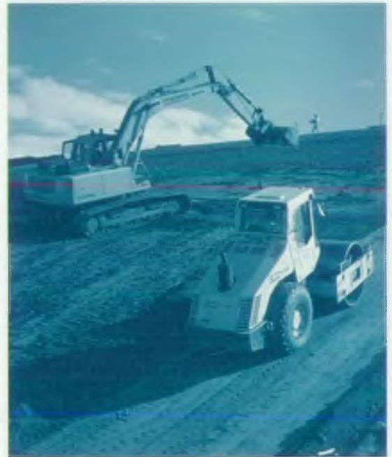
Site engineering to prevent pollution at a landfill site
