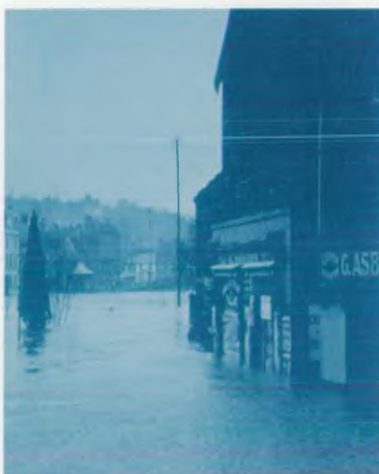
Flooding at Bewdley in the 1940s
