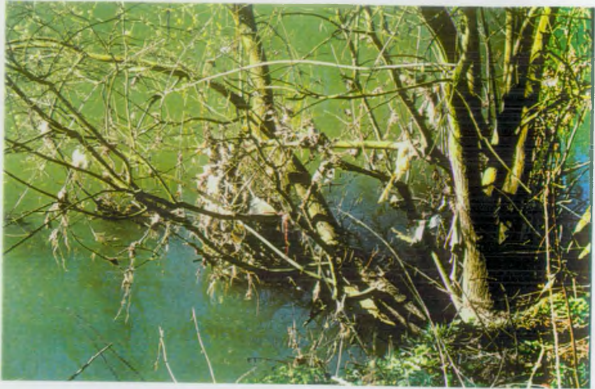
Photo 3 Close up of litter and sewage debris collected in branches of tree.
