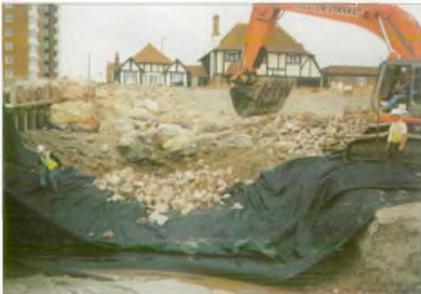
The area found to be at greatest risk was at Brooklands. As a result emergency work was put in hand during the summer of 1995 to reinforce the defences with 28,000 tonnes of shingle and the construction of three rock groynes to break up the wave energy and hold the beach in place.
