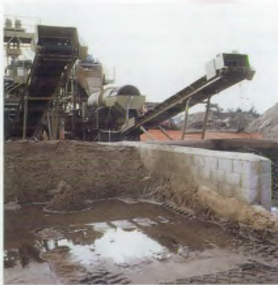
Top Basford gas works site, Nottingham - Receiving bunkers
