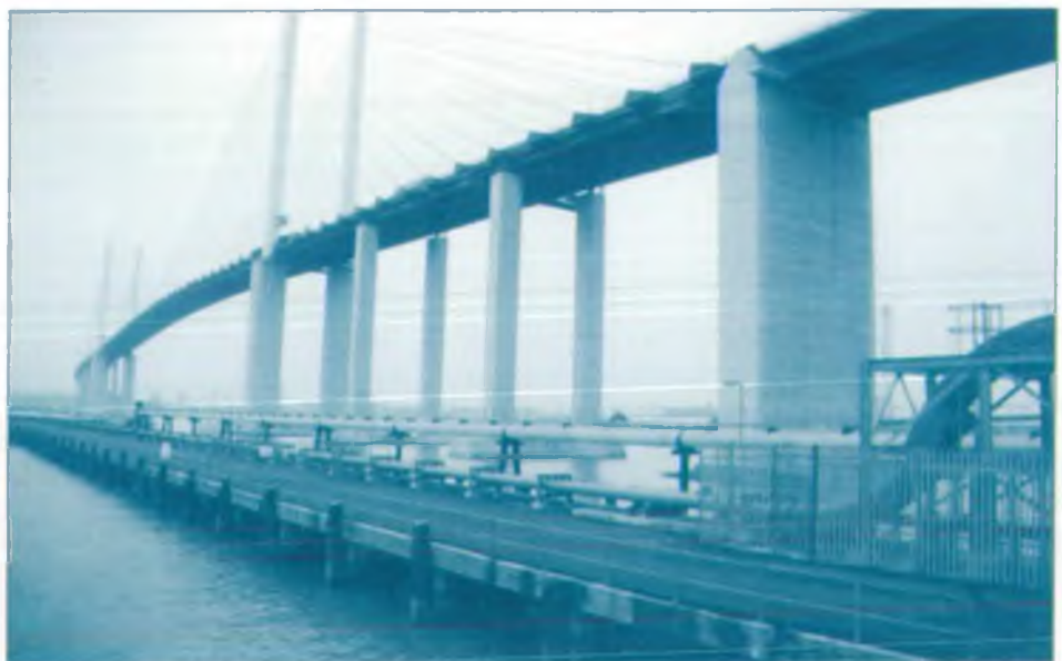
Queen Elizabeth II Bridge, Thurrock
