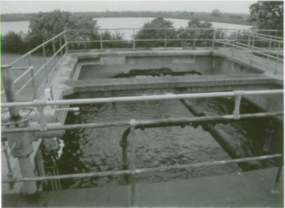
Hurleston Water Treatment Works
