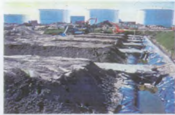
Treatment of contaminated soils in biopiles
