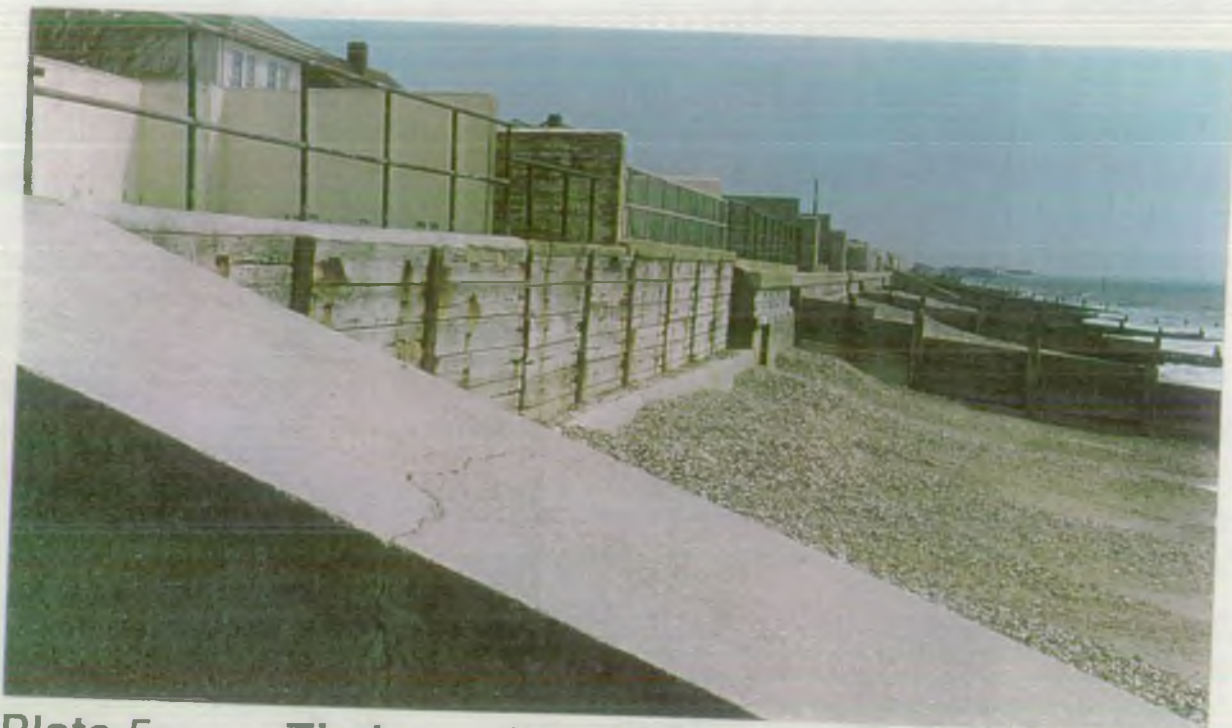
Plate 5 Timber breastwork along private frontages, East Wittering
