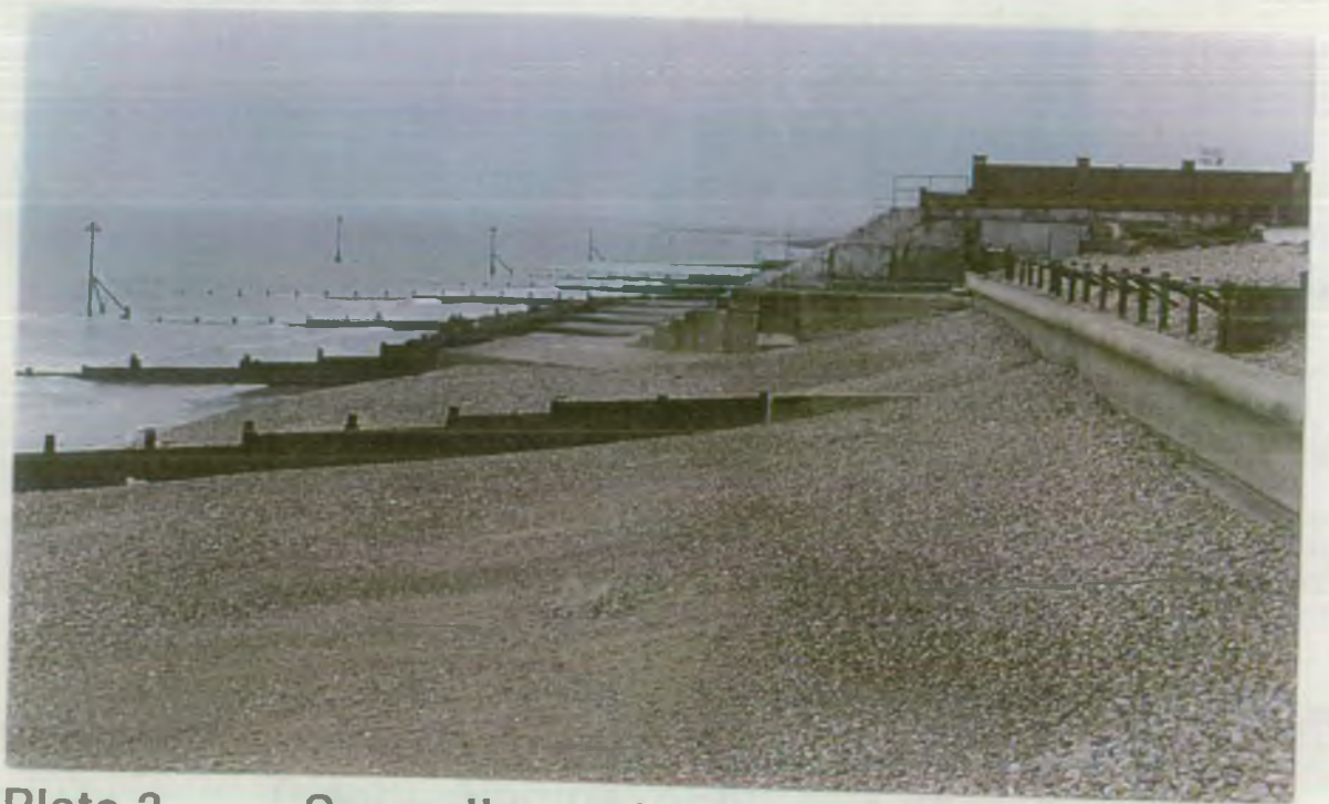
Plate 3 Seawalls and groynes, West Beach, Selsey
