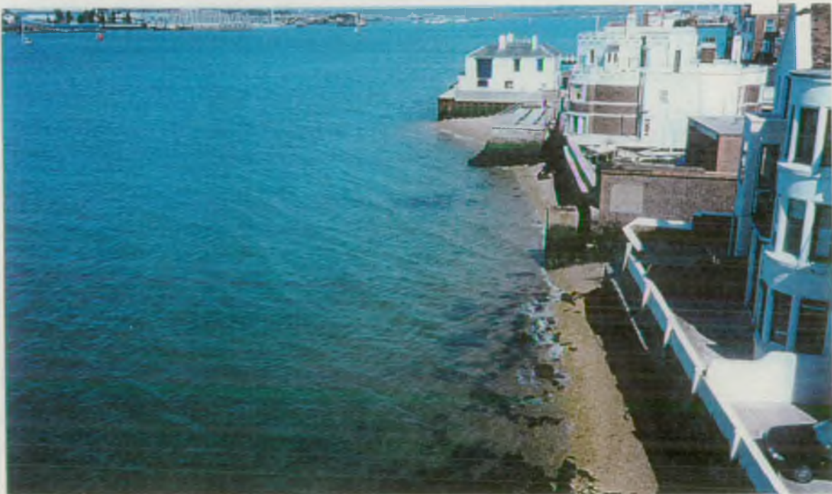
Plate 10 Defences at Portsmouth Harbour entrance, Old Portsmouth
