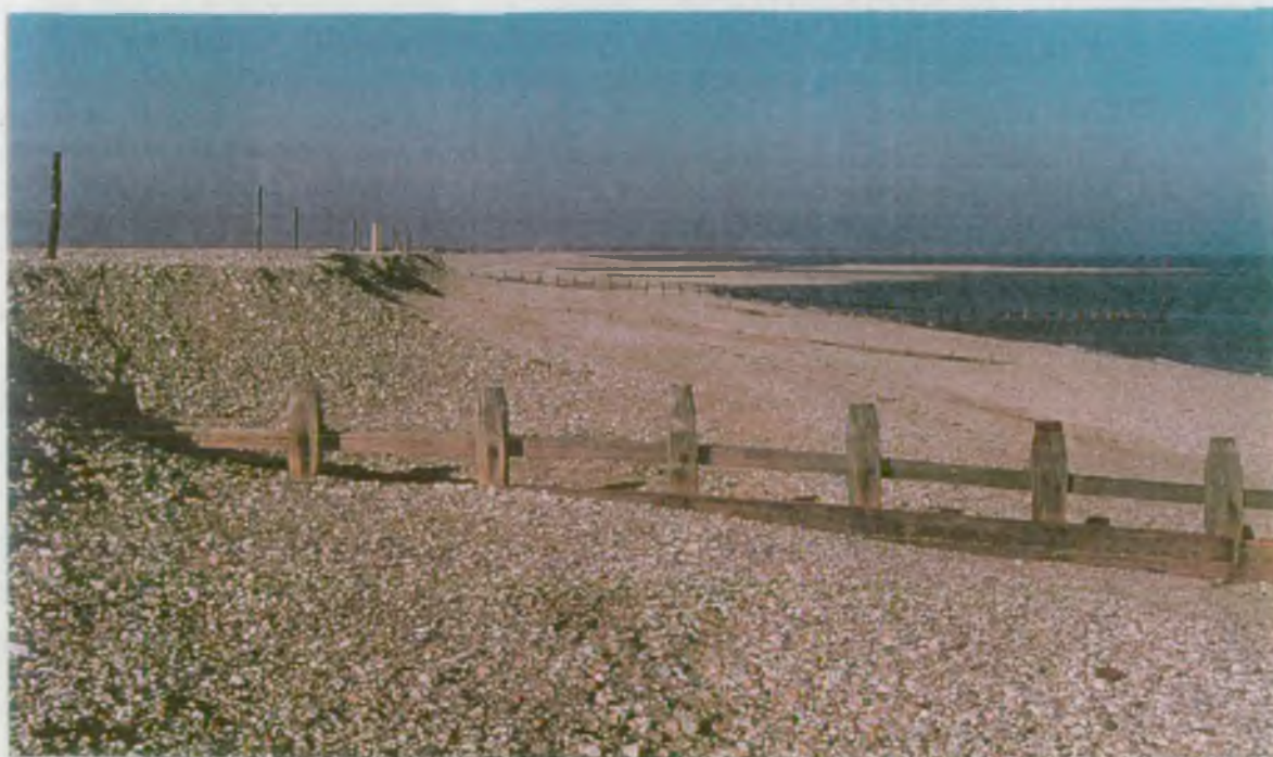
Plate 2 Timber groynes and low tide banks, south of Pagham Harbour entrance
