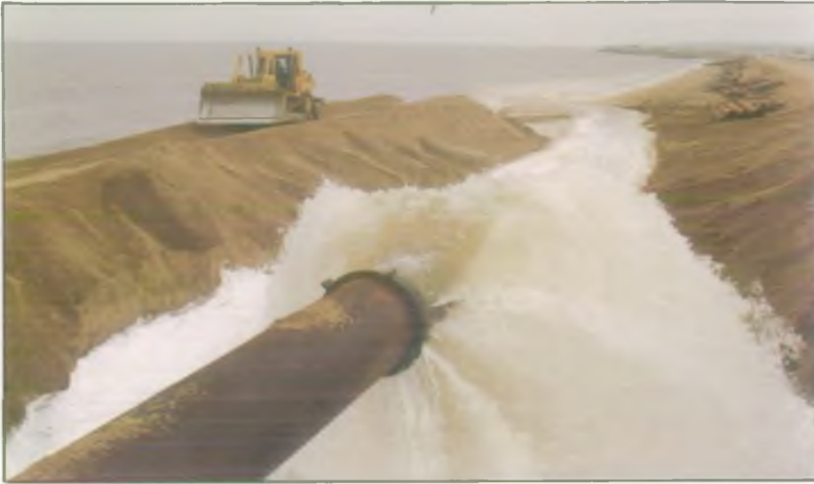
Heacham beach recharge in progress.
