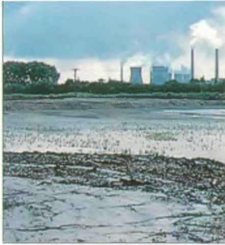
Pulverised fuel ash from power stations is deposited in sand and gravel excavations in the Trent valley.
