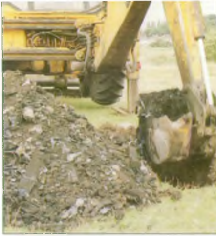
Trial pit investigation at a contaminated land site.
