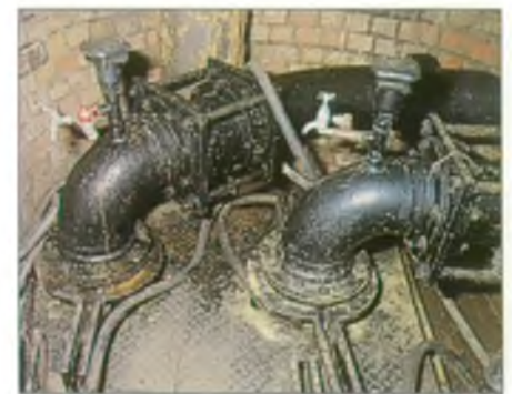
The top of a public supply borehole. Courtesy Severn Trent Water
