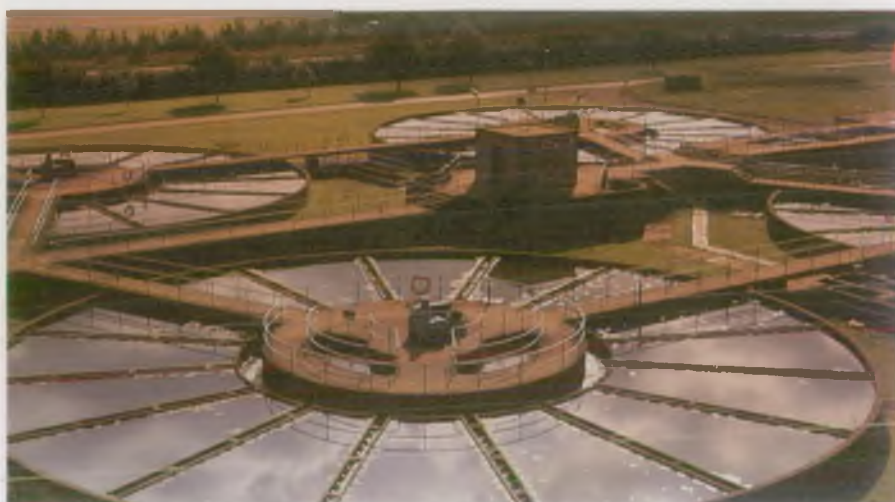
Huntington Water Treatment Works, Chester, supplies 400 megalitres (91 million gallons) of water every day.
