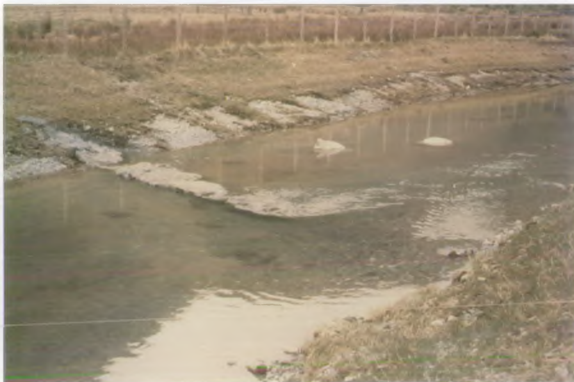
Figure 23 Habitat Improvement by Groyne Construction
