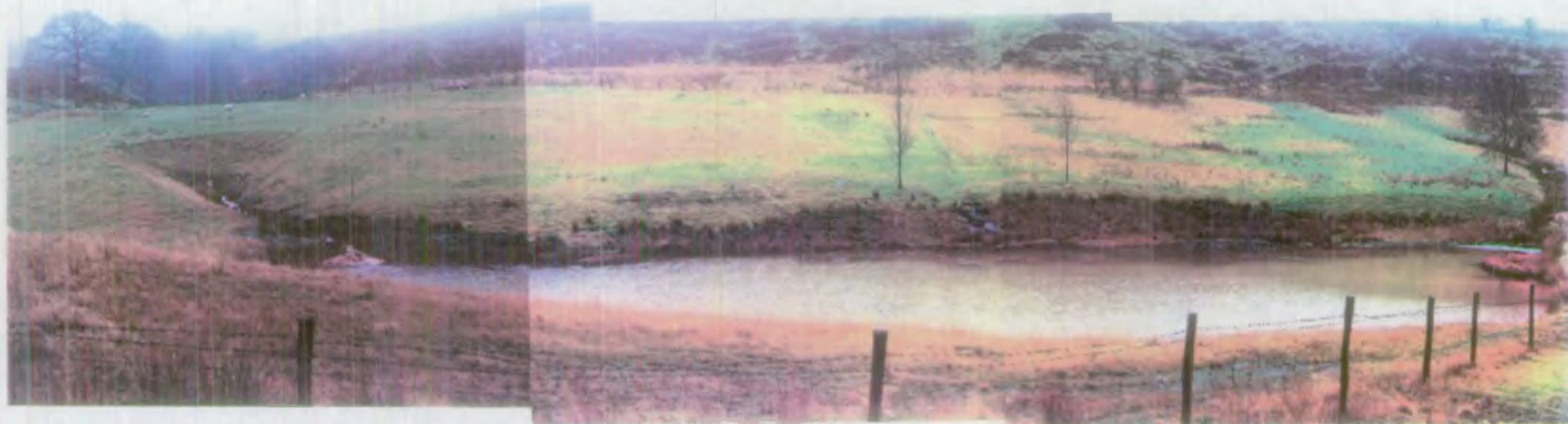
The Whitworth Lagoon. Whitworth A enters from the left, Whitworth B from the right. The drainage ditch from the road is clearly visible in the centre.
