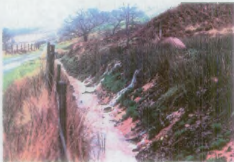
Gwenffrwd discharge entering recently constructed channel.
