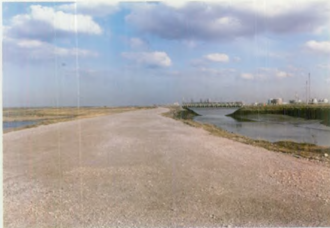
DOUBLE BAILEY BRIDGE CARRYING EMERGENCY ACCESS ROAD - MARCH '95 VIEWED FROM NORTH BANK EAST
