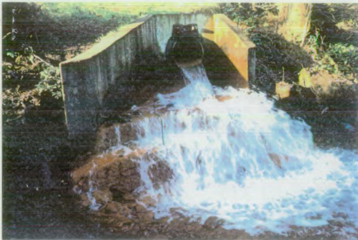
Ferruginous minewater discharge to the R. Sirhowy (6) at Pontllanfraith.
