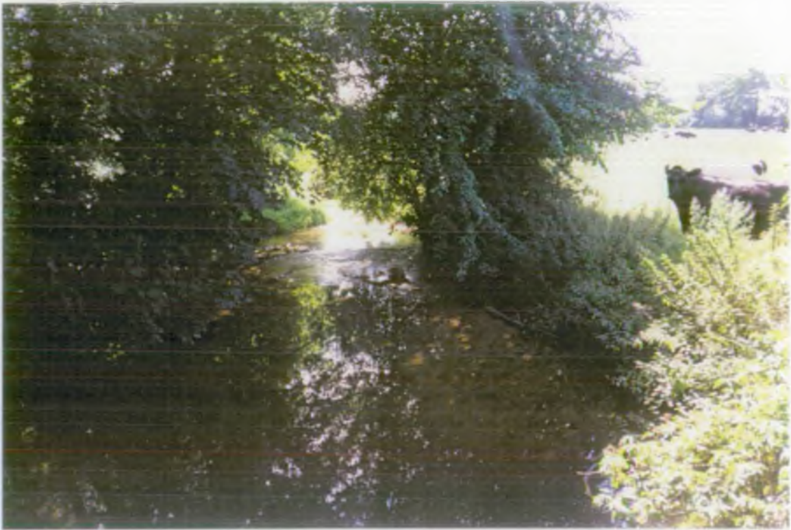
PHOTO 5 - Downstream view from footpath bridge. Grid Ref. (0980,9616).
