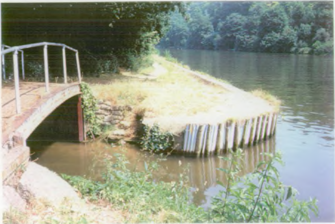
PHOTO 1 - Start of White Brook at outlet from River Thames. Grid Ref. (9054,8327).
