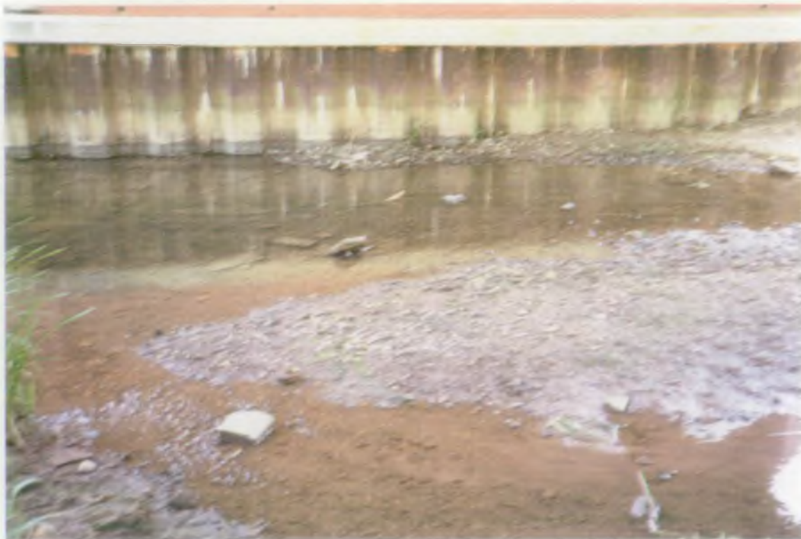
PHOTO 5 - Low water flow and building material in stream. Grid Ref. (4592,4167).
