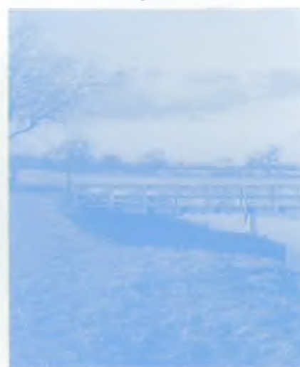
Merron's Bridge at high tide
