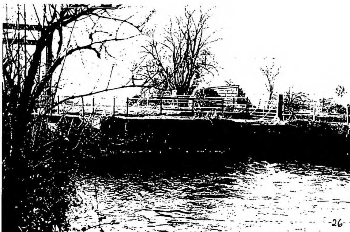
Stanwick Sluices - viewed from downstream
