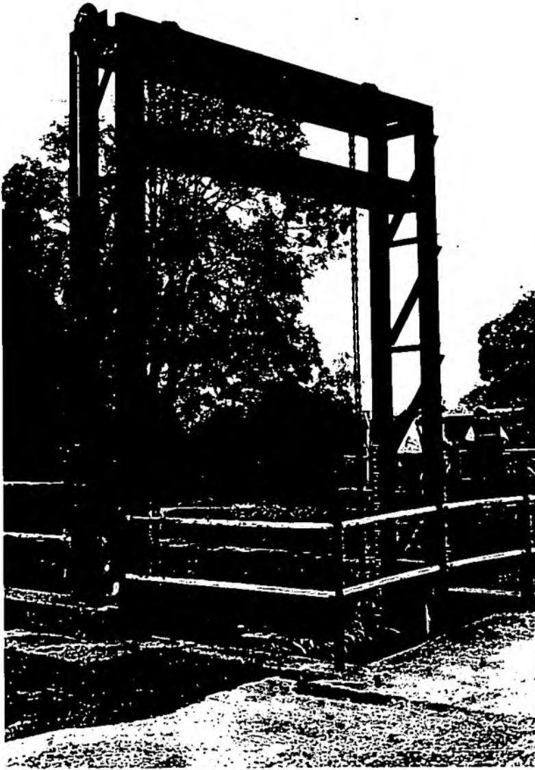
Stanwick Vertical Gate Sluice
