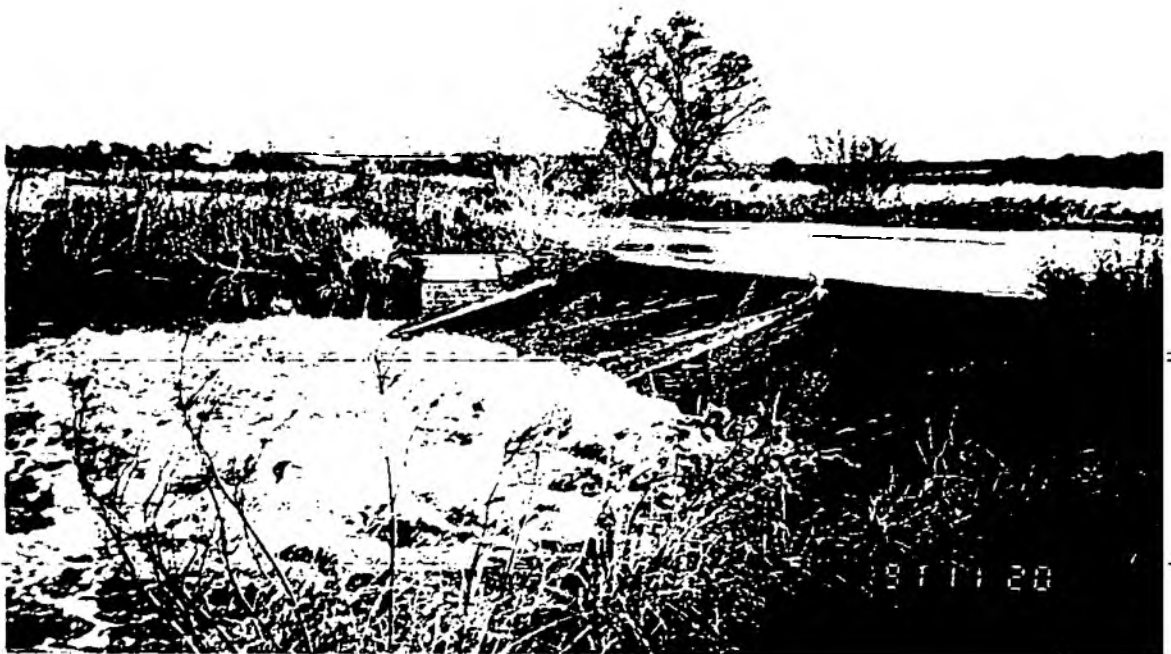
Weir No. 1 - high river flows on 20.11.91
