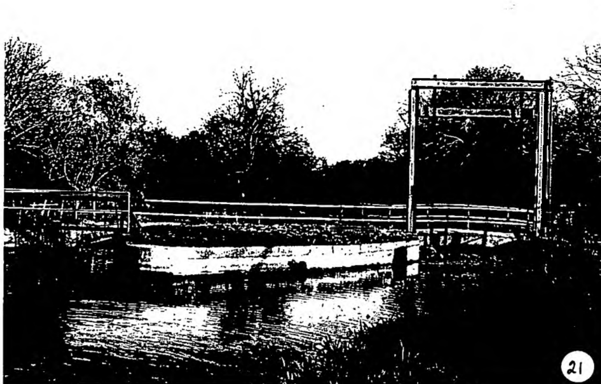
Stanwick Sluices - viewed from upstream
