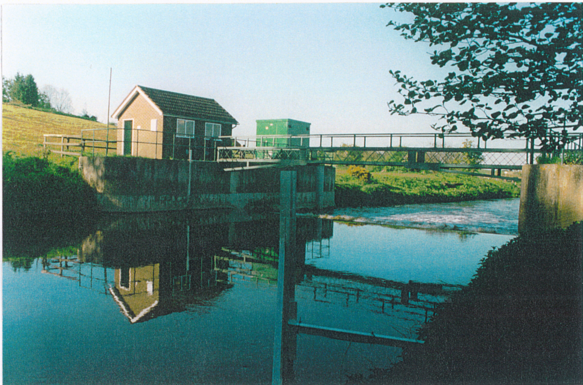
View downstream and across to the Walcot gauging station and weir from the upstream transducer rack, visible in the immediate foreground.
