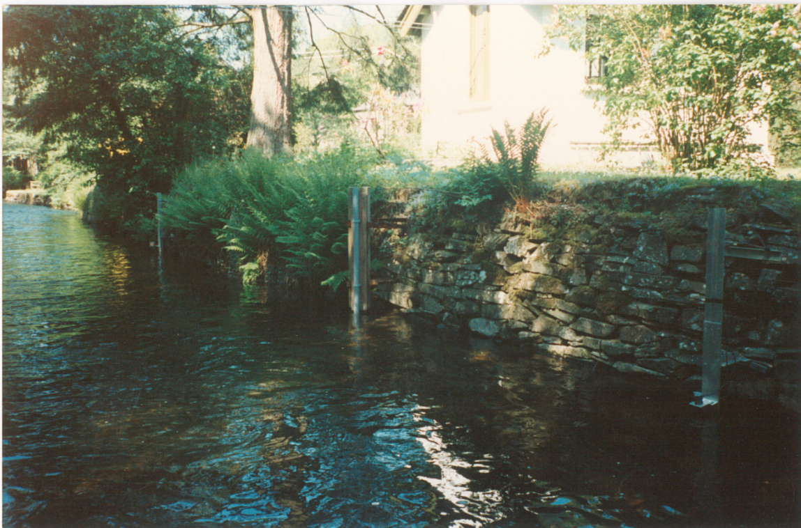
Low Nibthwaite - view upstream to near bank showing the two transducer racks together with the depth mounted in the stilling tube.
