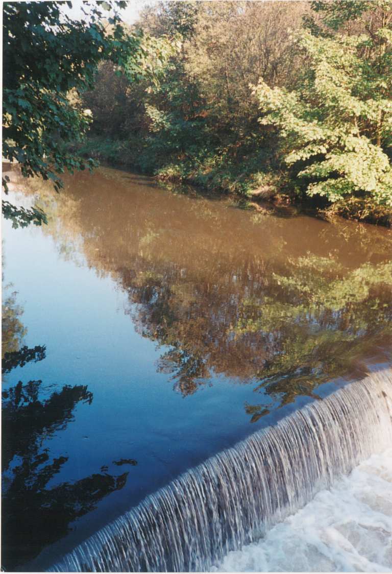
Blackford Bridge weir under low flow conditions
