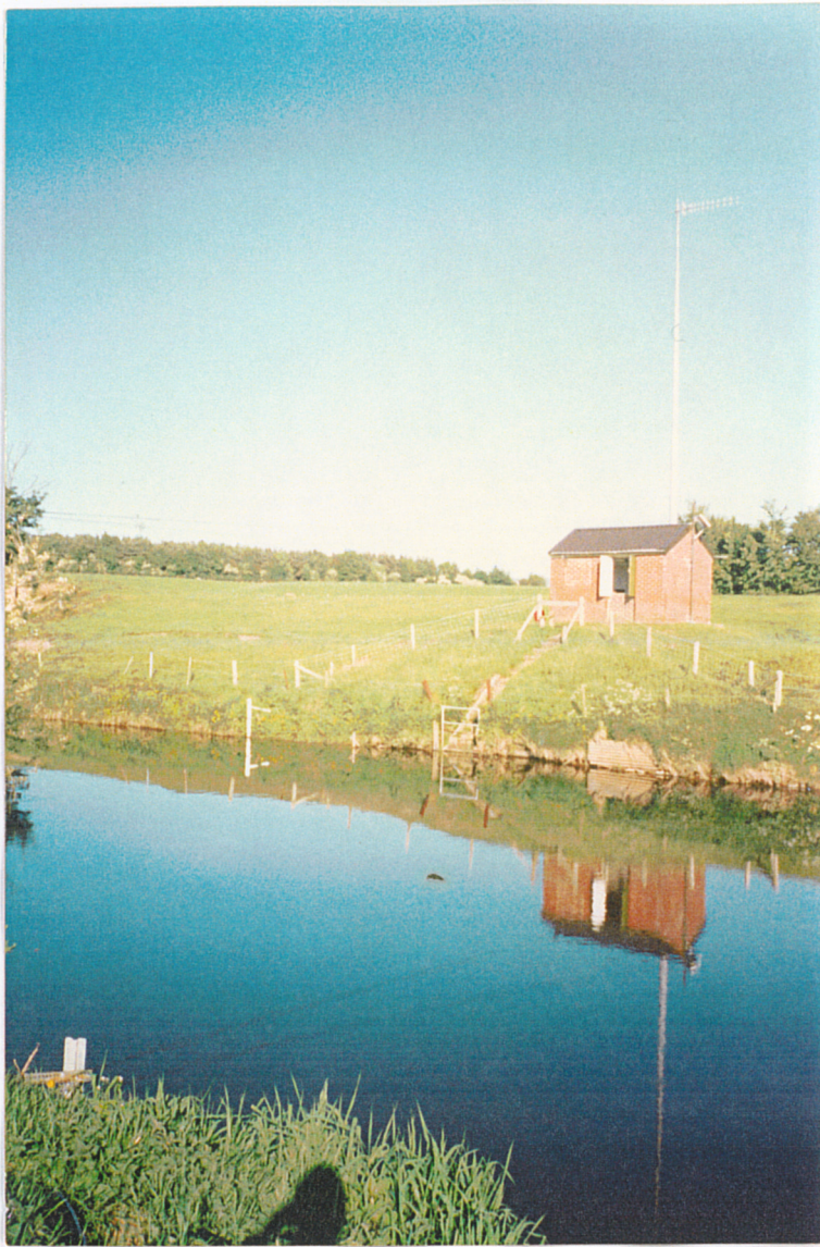
Looking across to the Greenholme station hut along the line of the velocity paths. Transducer racks can be seen in the immediate foreground (downstream) and on the far bank (upstream).
