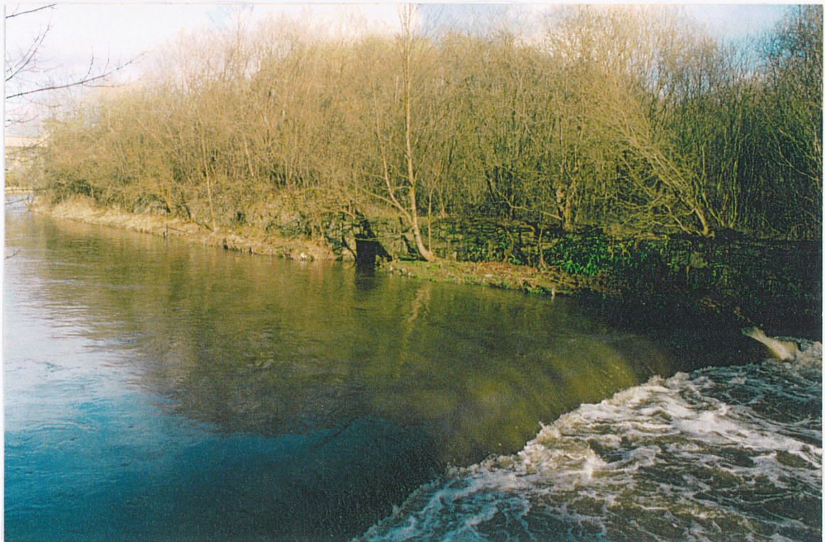
Blackford Bridge weir and channel under high flow conditions
