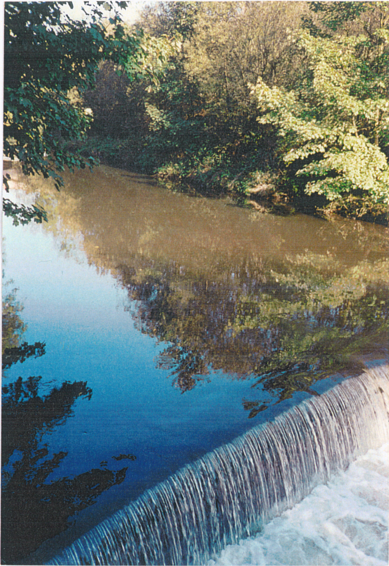
Blackford Bridge weir under low flow conditions
