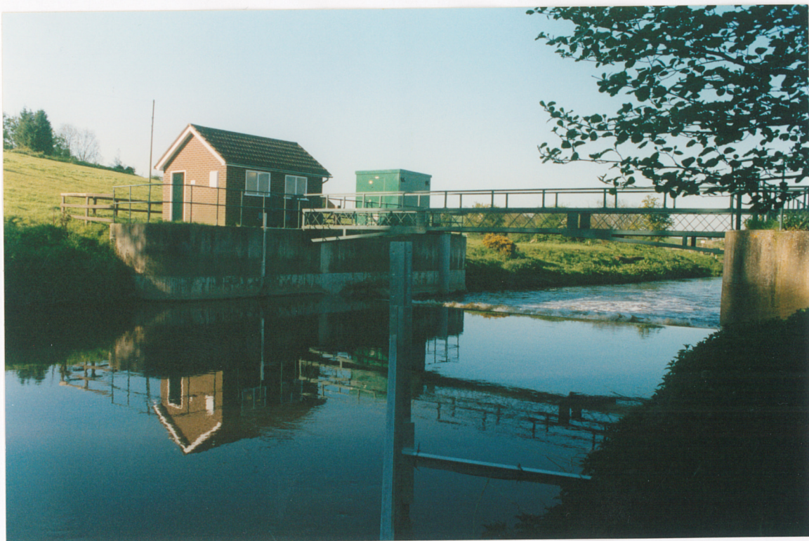
View downstream and across to the Walcot gauging station and weir from the upstream transducer rack, visible in the immediate foreground.
