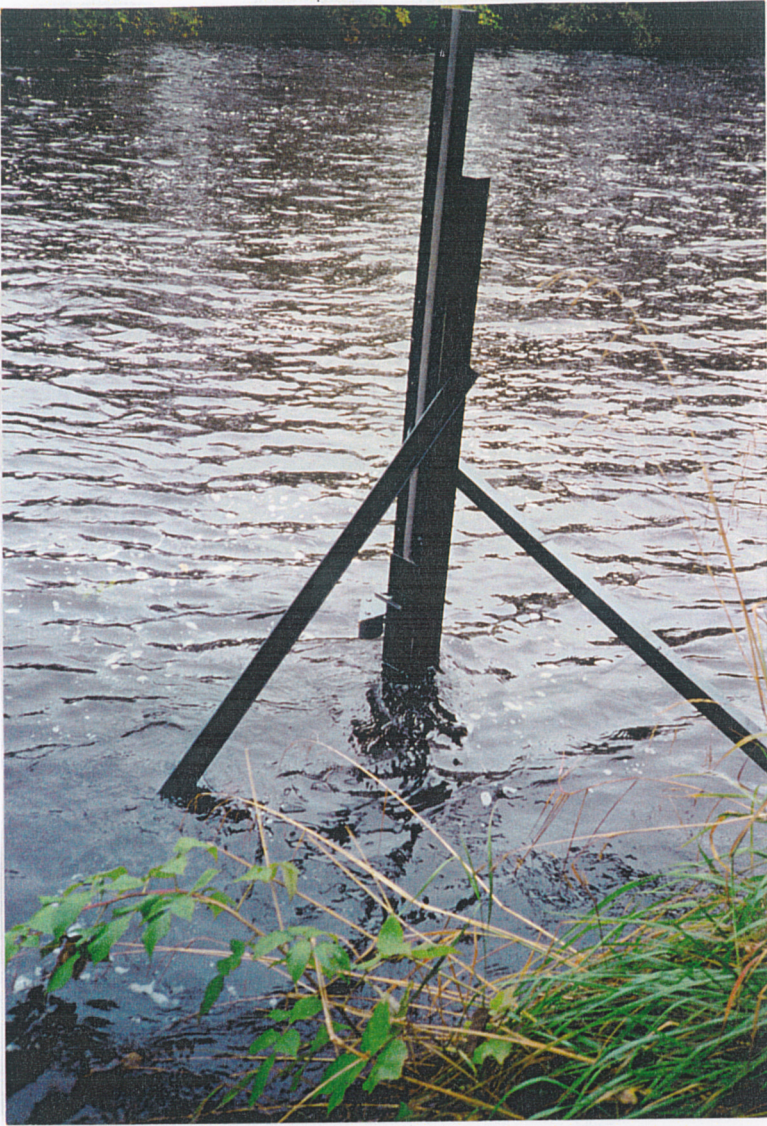
Close up of upstream transducer rack at Middleton in Teesdale
