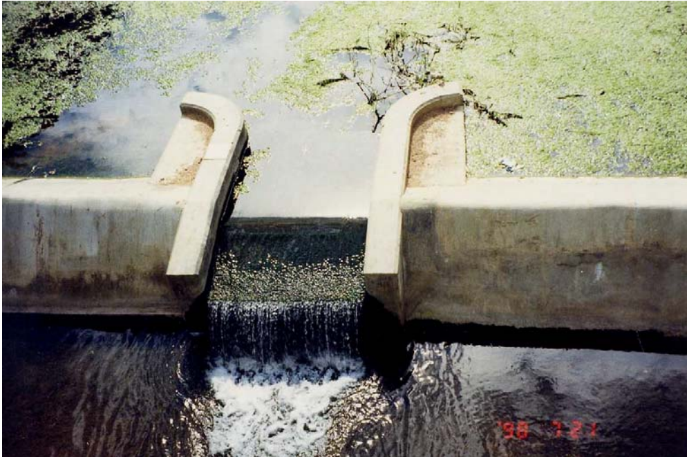
Figure AD9 - Weir with low flow notch
