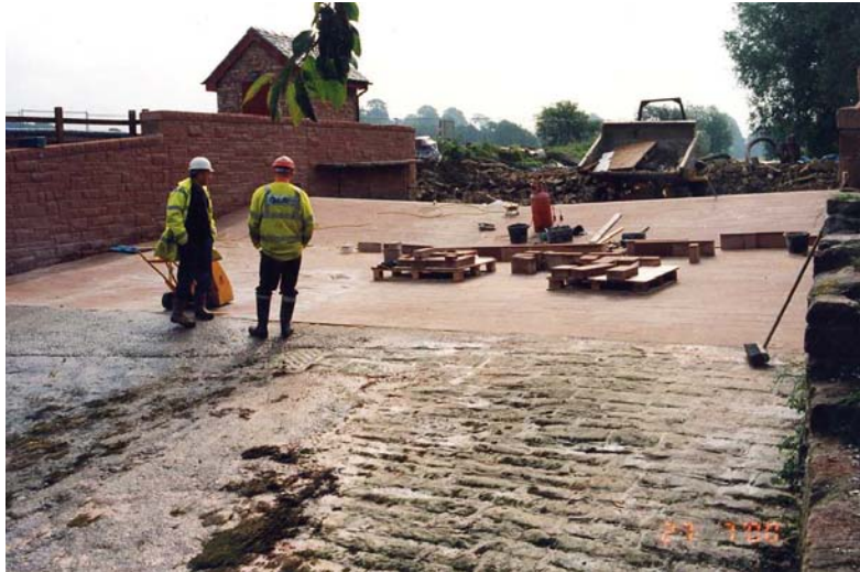
Figure M4 – The new weir crest neatly joining the existing glacis
