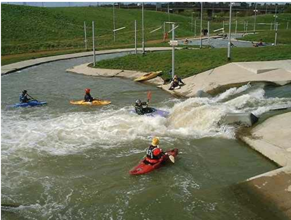
Figure AD10 - Variable configuration weir at the Nene White Water Centre, Northampton
