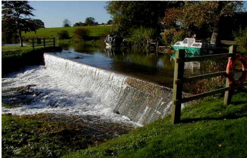
Figure 2.6 Dangerous side weir?
