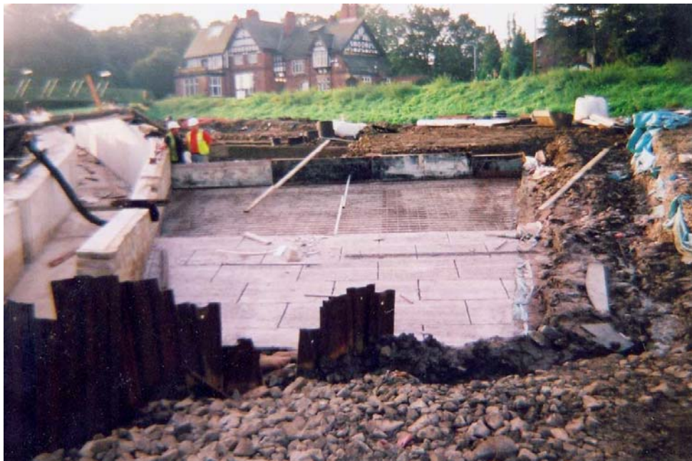
Figure L3 – New weir taking shape adjacent to the fish pass
