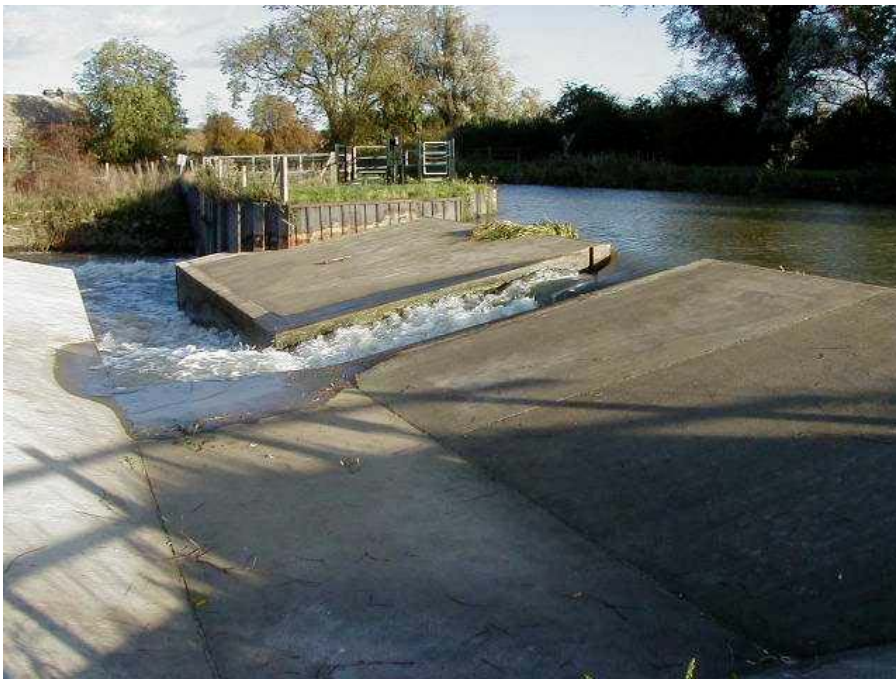
Figure AD4 - Side weir with fish pass
