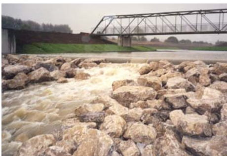
Figure F3 – View of the new weir in operation
