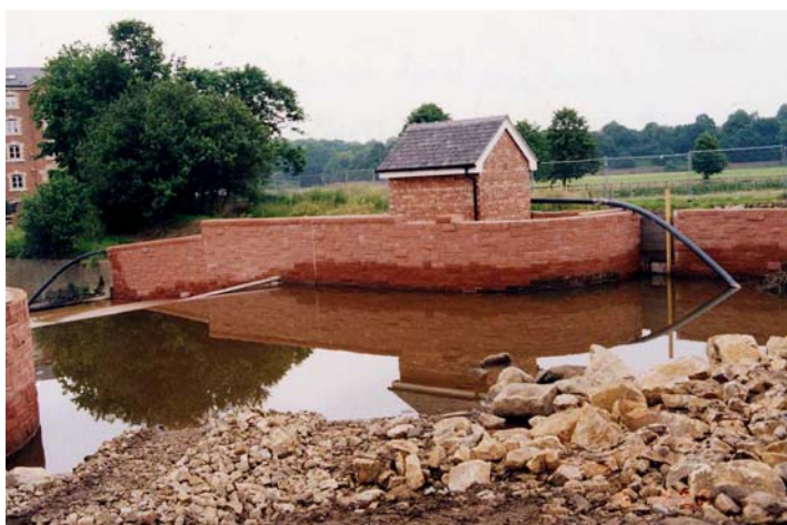
Figure M6 – Completed wall and instrumentation building
