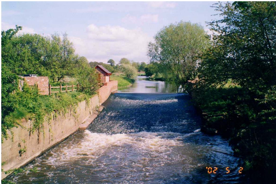
Figure M7 – The completed weir
