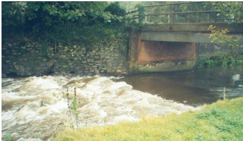
Figure C4 - View of the site in October 2002 with bed remaining stable
