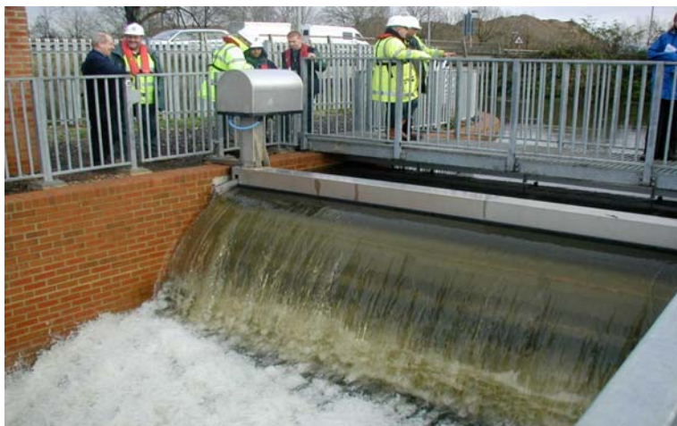
Figure 2.13 Aerated nappe
