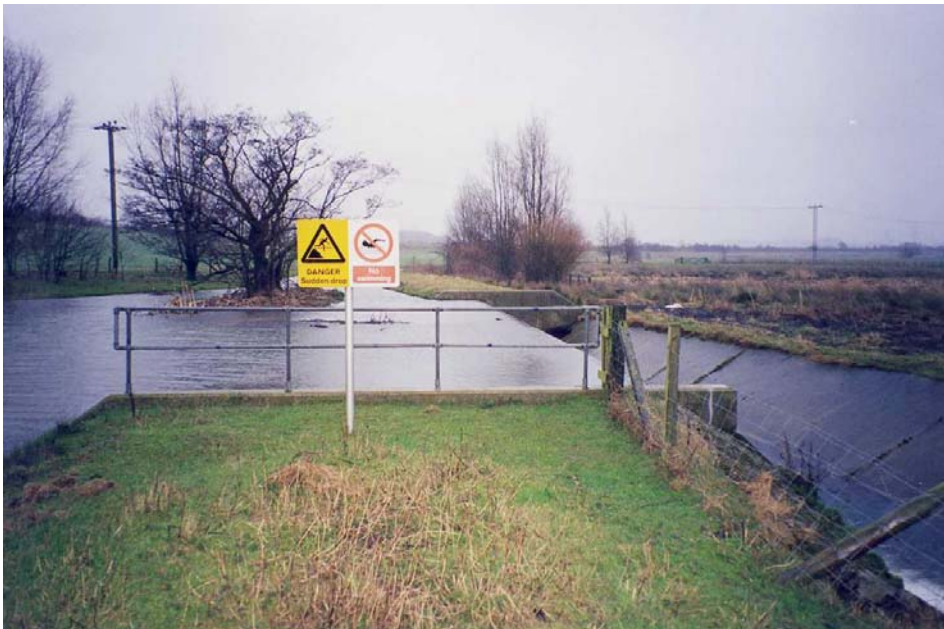
Figure AD8 - Warning sign and fencing
