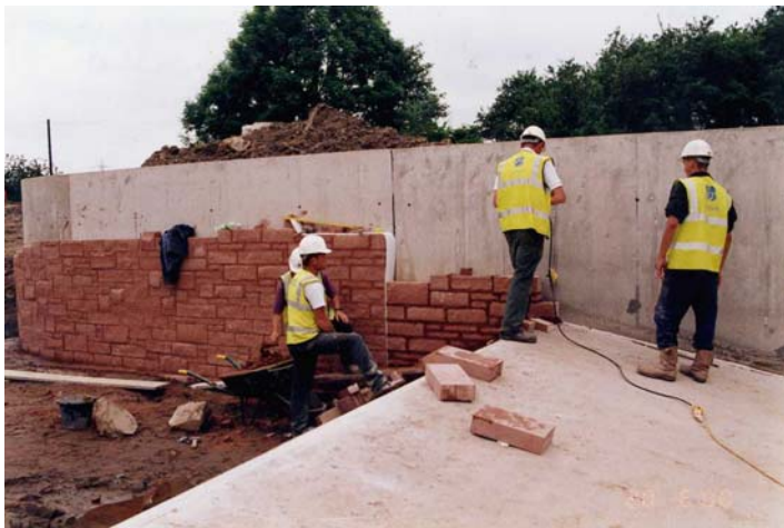
Figure M5 – Stone facing to the concrete walls
