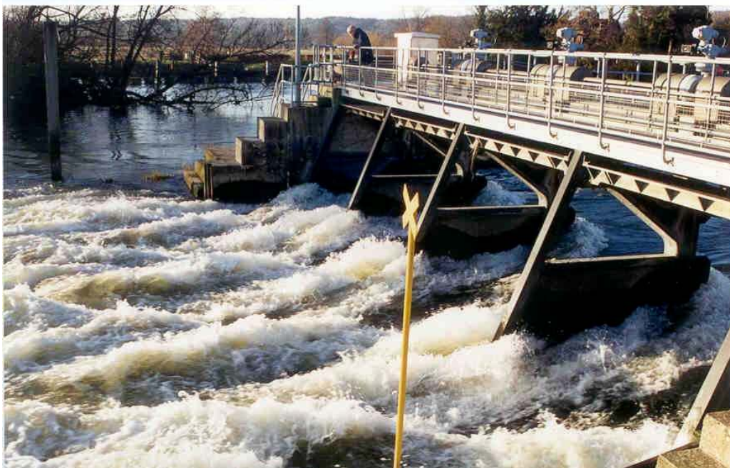
Figure H1 – Before addition of the of the “kicker” devices
