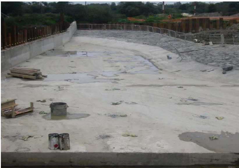
Figure K3 – The left-hand half of the weir from downstream.
