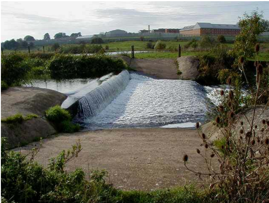
Figure AD6 - Weir with ford
