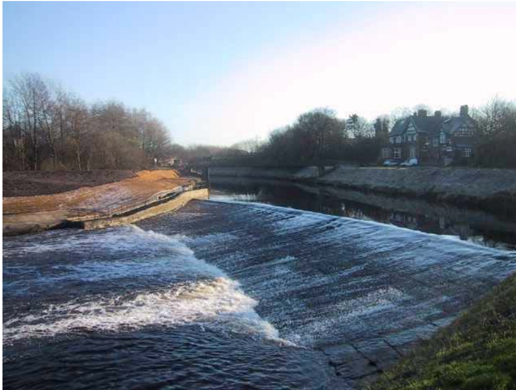
Figure L4 –Completed weir structure with the new fish pass on the far bank
