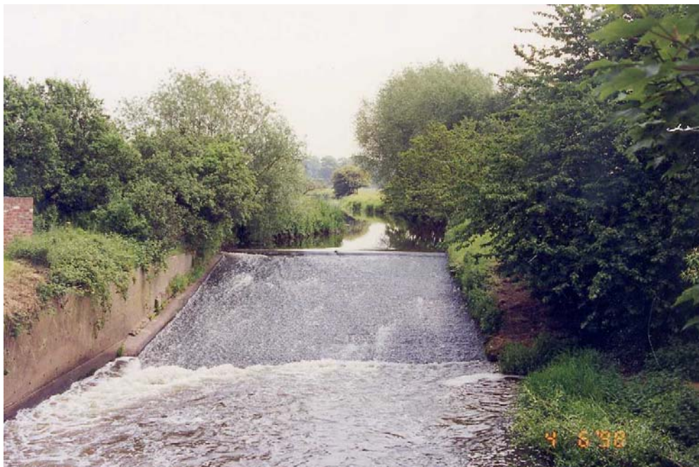
Figure M1 – The weir before the works were carried out
