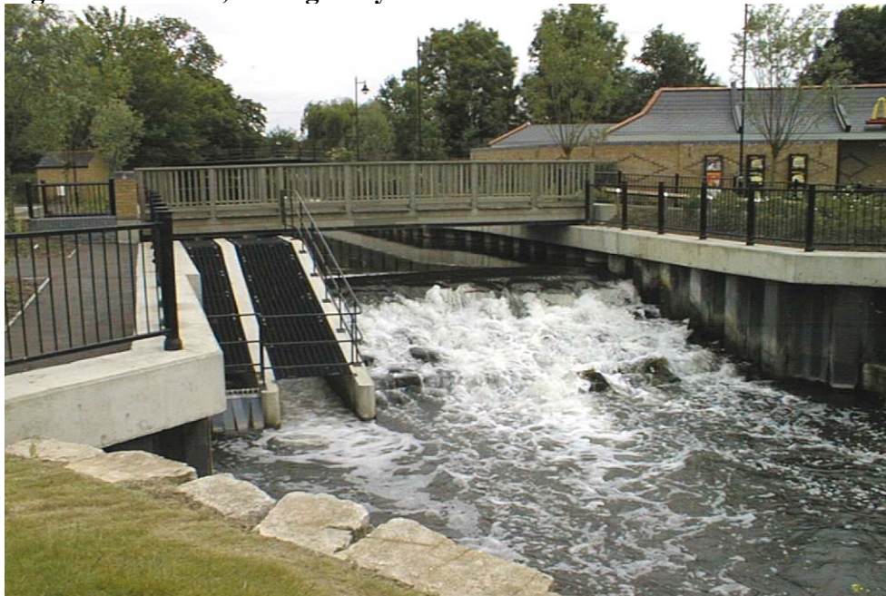
Figure N2 – Weir, with corrected flow
