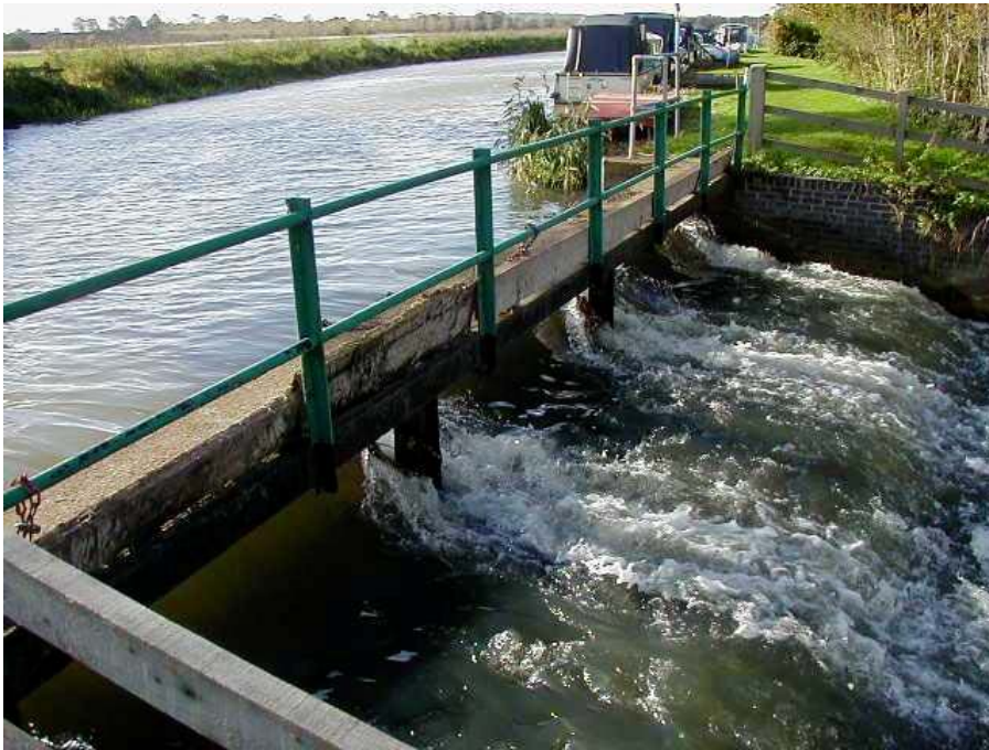
Figure AD3 - Side weir with narrow footbridge
