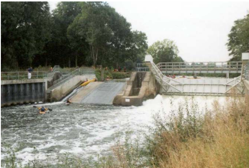
Figure 2.30 Weir with a canoe pass on the River Medway
