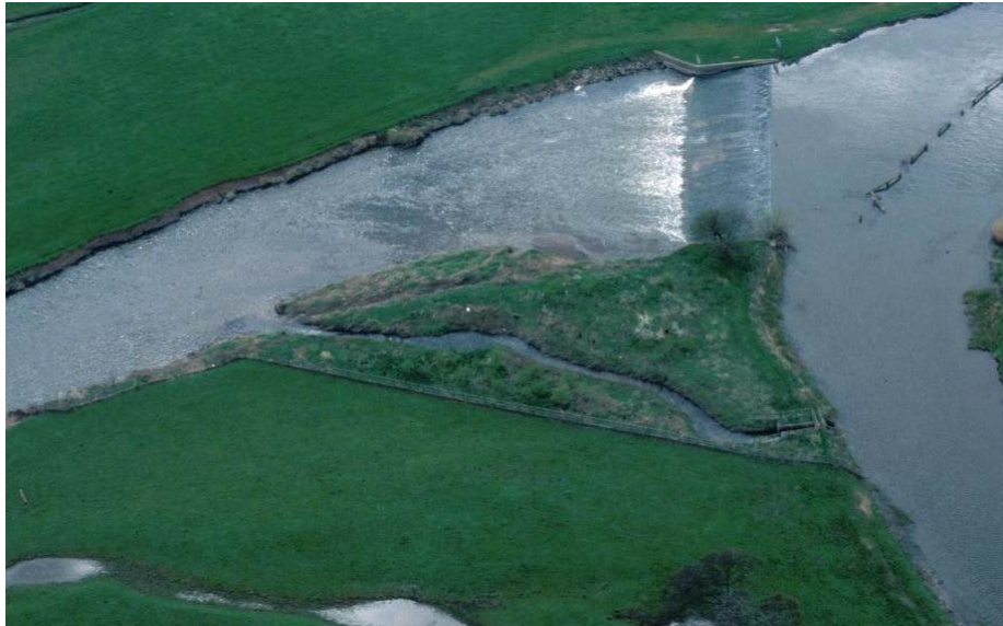
Figure A5 - Aerial photograph of finished channel
