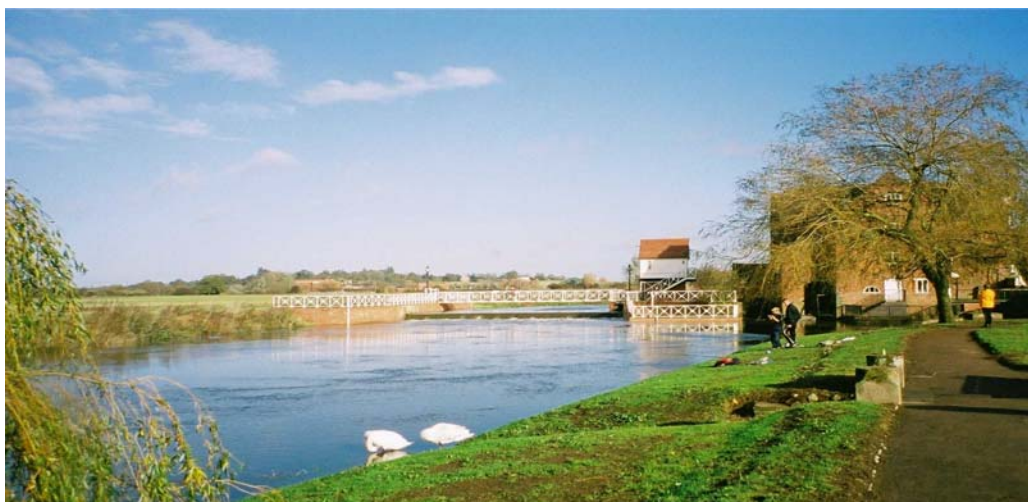
Figure 1.2 Tilting gate weir at Tewkesbury
