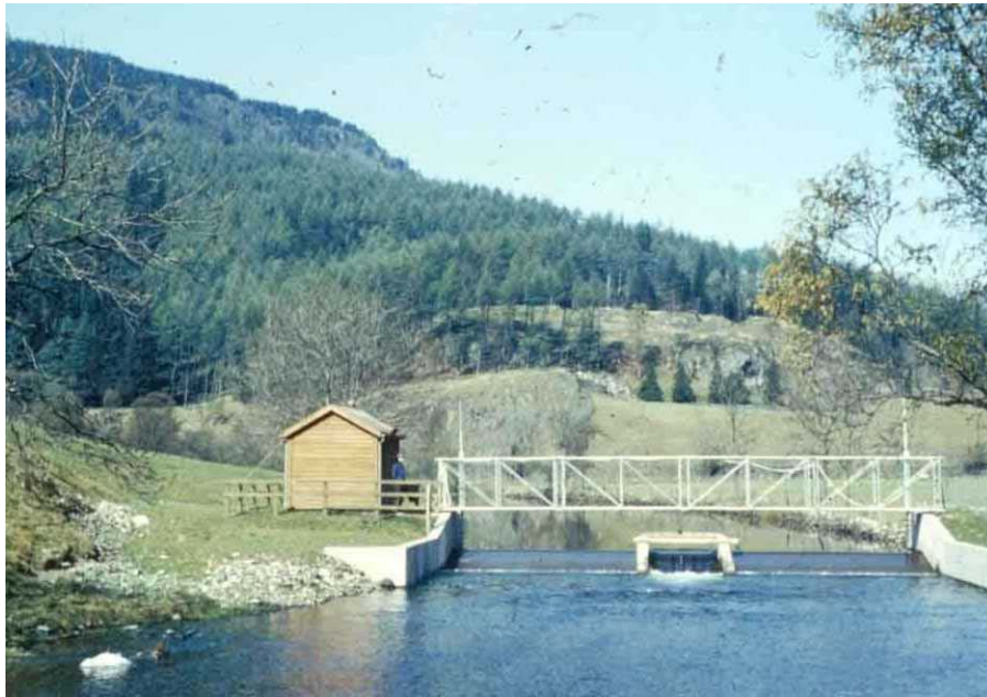
Figure 2.11 A flow gauging weir with a central low-flow section
