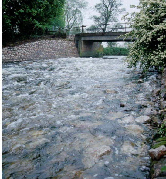
Figure C3 - Completed rock chute with rebuilt bank protection
