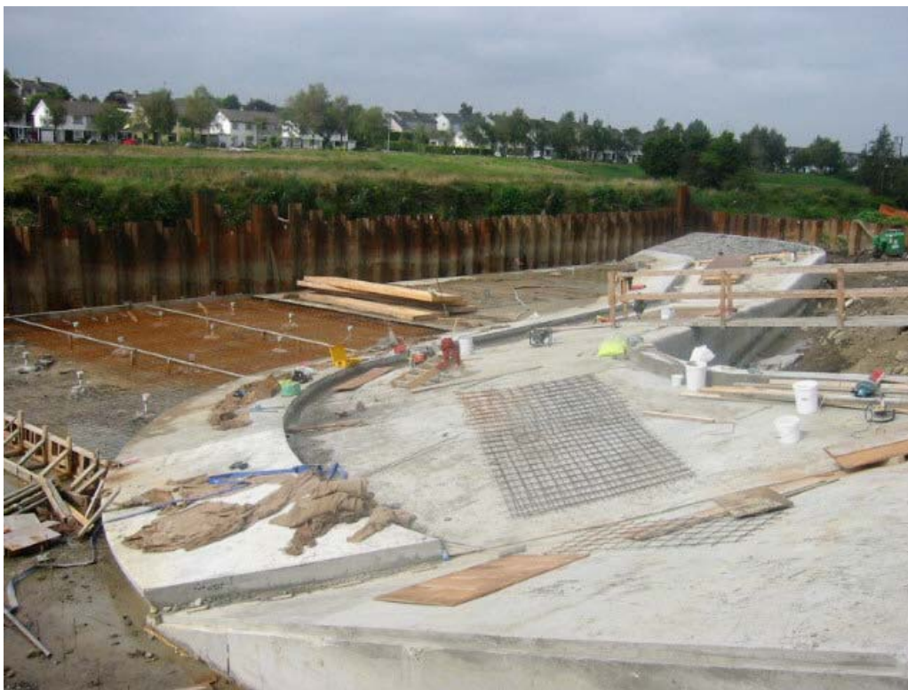
Figure K1 – The first half of the weir under construction.
