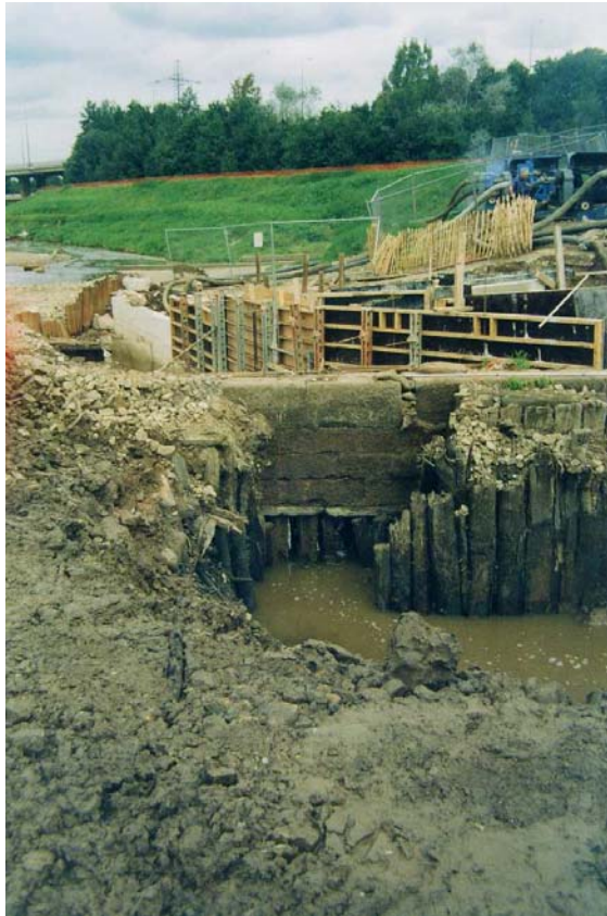
Figure L2 – Excavation reveals the timber piled sub-structure
