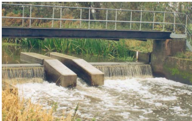
Figure D1 – The original weir with its new fish pass
