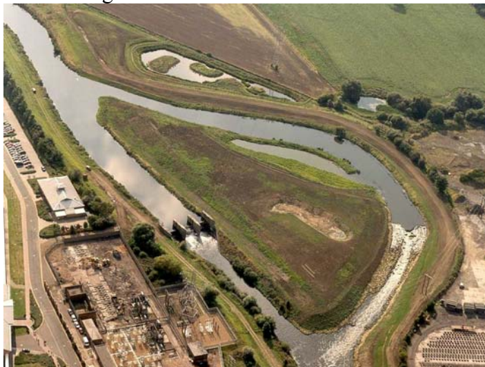
Figure B5 - View of the finished works
