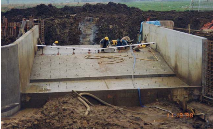
Figure 2.12 Construction of crest for a flow gauging weir
