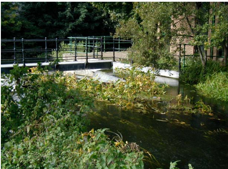
Figure 1.9b The same weir with weed growth
