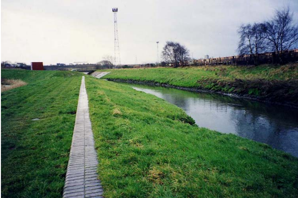
Figure AD1 - Grassed side weir
