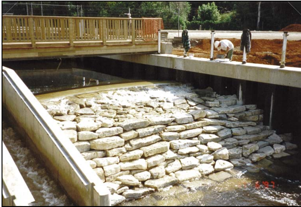
Figure N1 – Weir, as originally constructed
