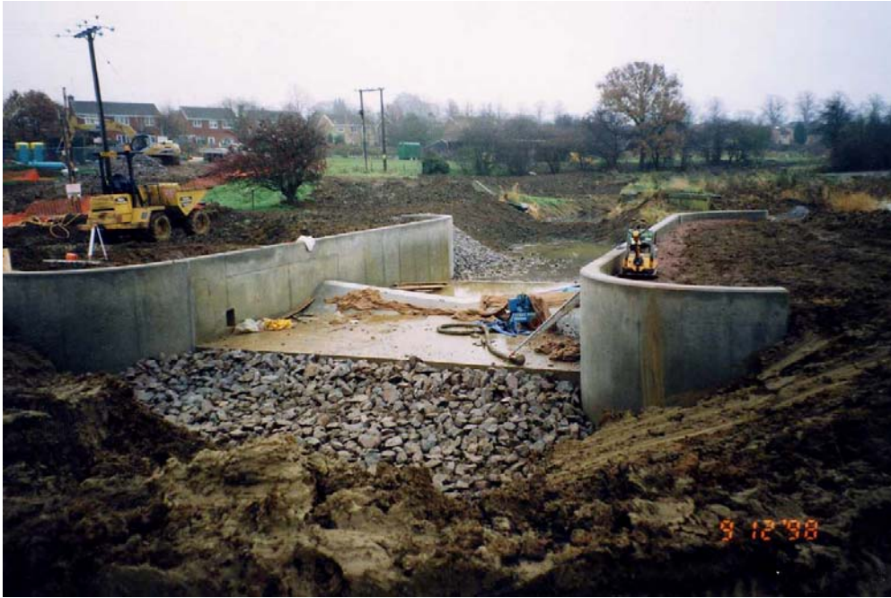
Figure AD7 - Construction of a flat-vee weir
