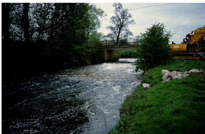
Figure C2 – The completed rock weir in operation
