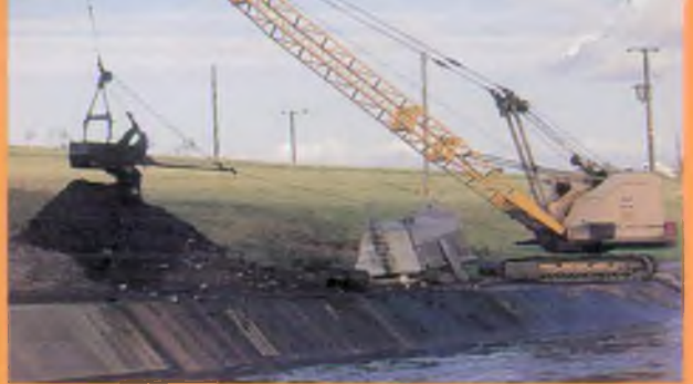
Bank work on the River Tame
