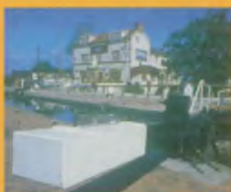
The lock at Beeston Weir, where the Beeston Canal joins the Trent
