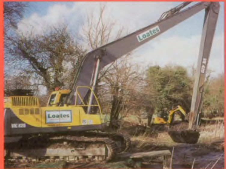
Removing silt from the lake
