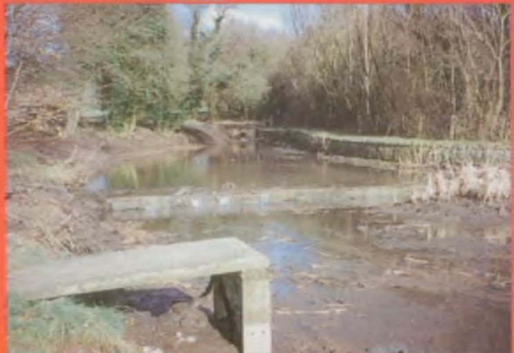
The silt trap is exposed as work nears completion
